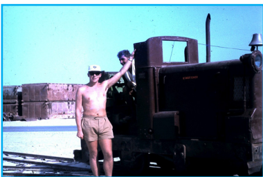
Re-building The Railway
